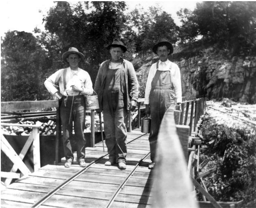
Workers stand on a tramway near the top of a lime kiln (back left) in Johnson, 1900s-1910s. Marion Mason, photographer/Philip Steele Collection
